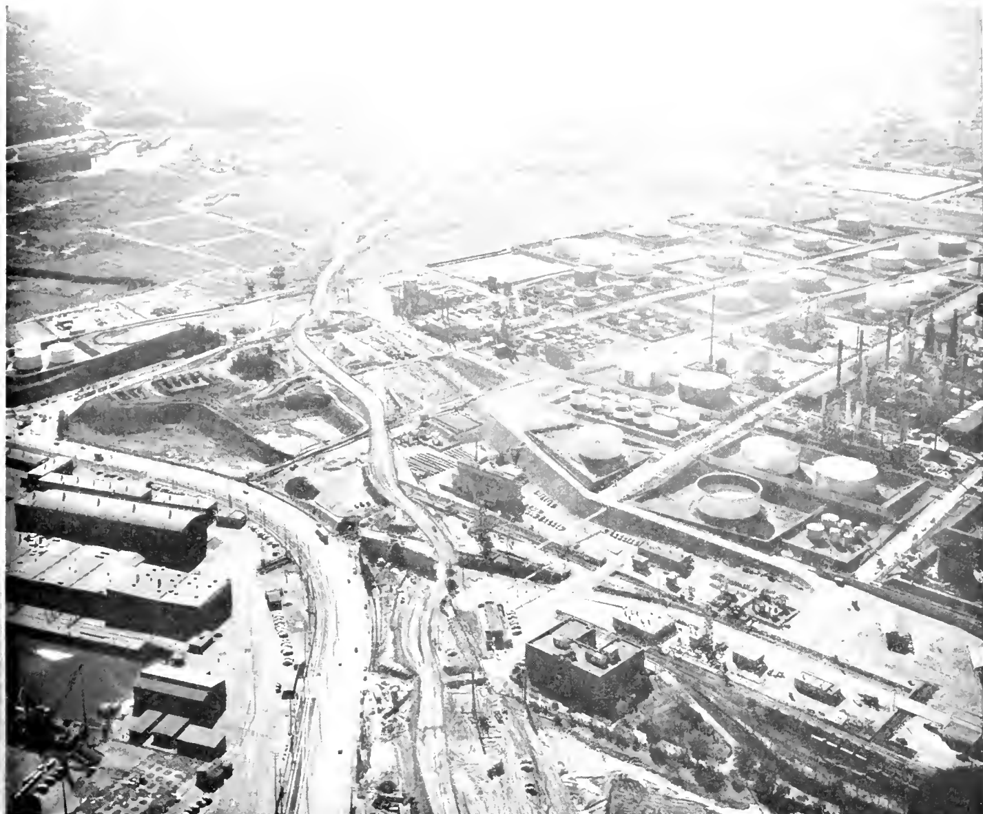
Aerial view looking southerly of excavation area and haul road through oil refinery. At left is Wilmington-San Pedro Road. Traffic artery shown in background is Gaffey Street extending into San Pedro.
